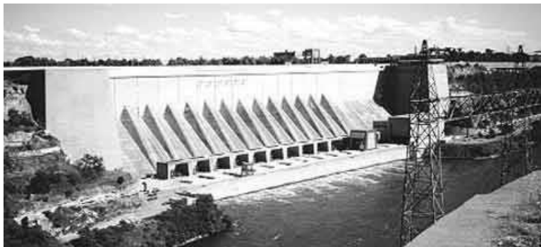
Figure 8.3: The Ontario Power Generation station
